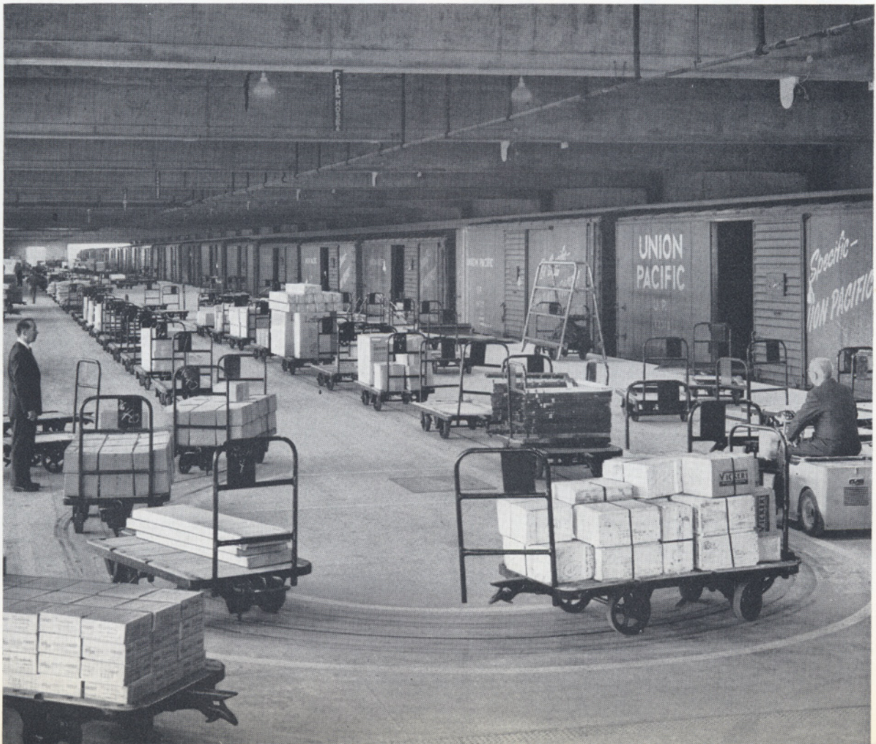
Interior of new freight house, East Los Angeles.
