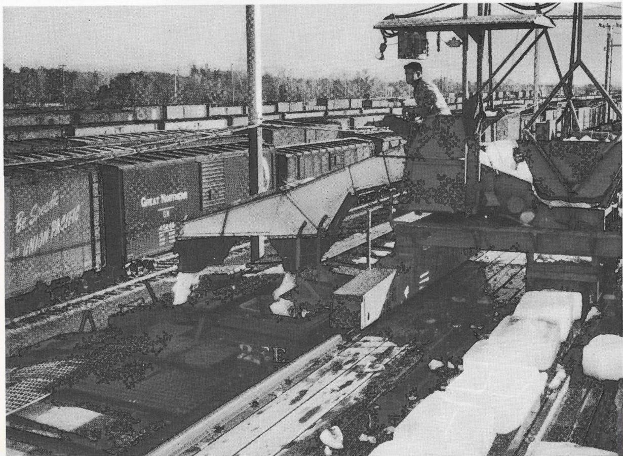
Pacific Fruit Express icing machine facilities in use at Ogden, Utah.
