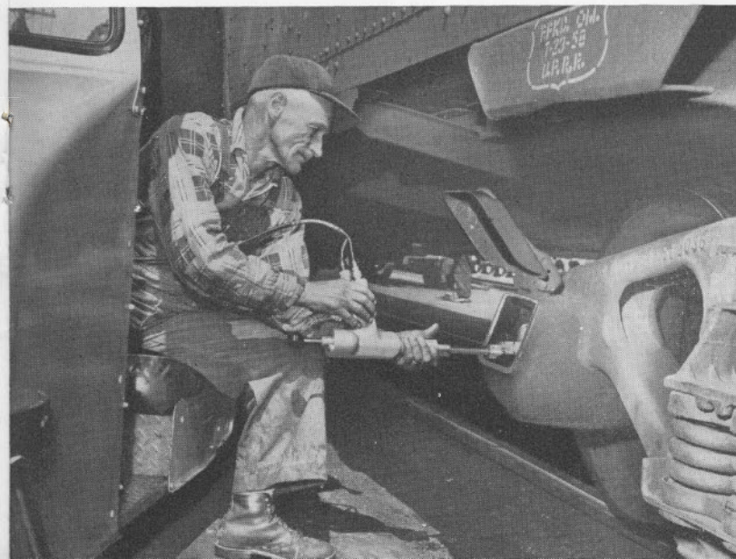
The Sperry Reflectoscope, an ultrasonic device applied to journals, locates axle defects instantly and shows them on a screen in a manner similar to television.
