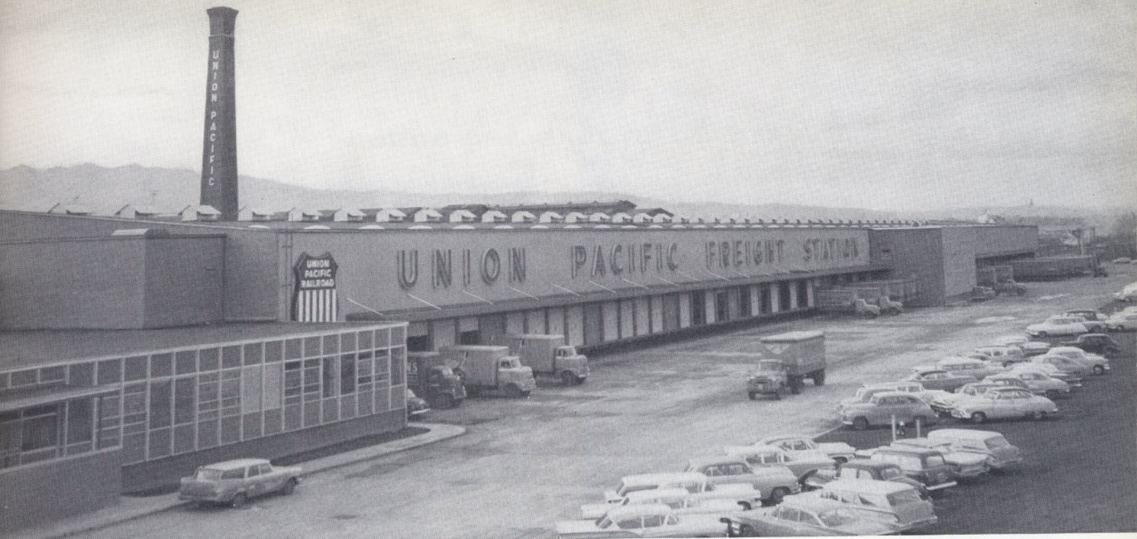
New Freight House at the enlarged and modernized Albina Yard, near Portland, Oregon.
