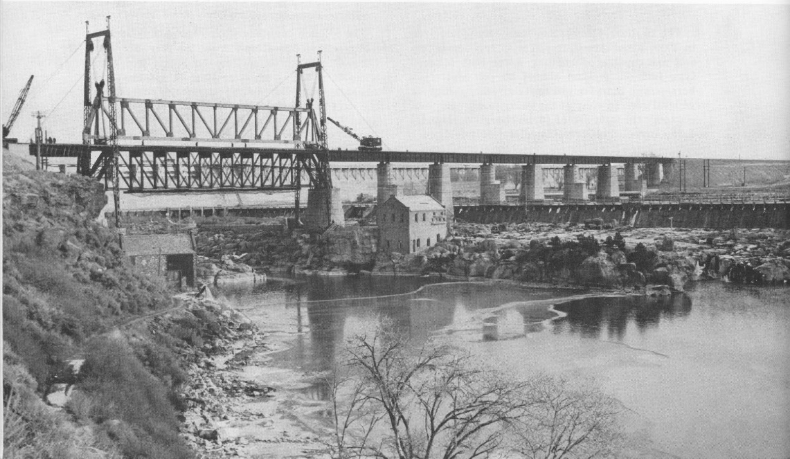
New truss for the American Falls Bridge about to be lowered into position.
