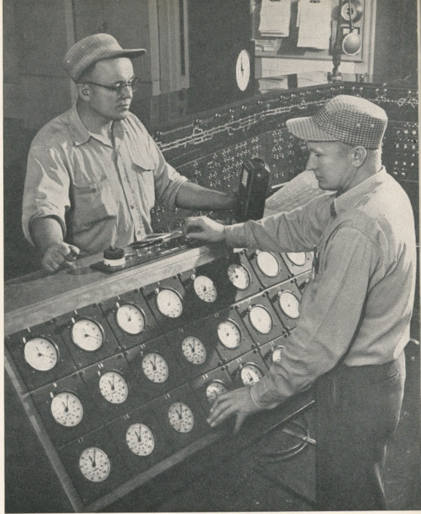
Installing CTC equipment at Pocatello, Idaho.
