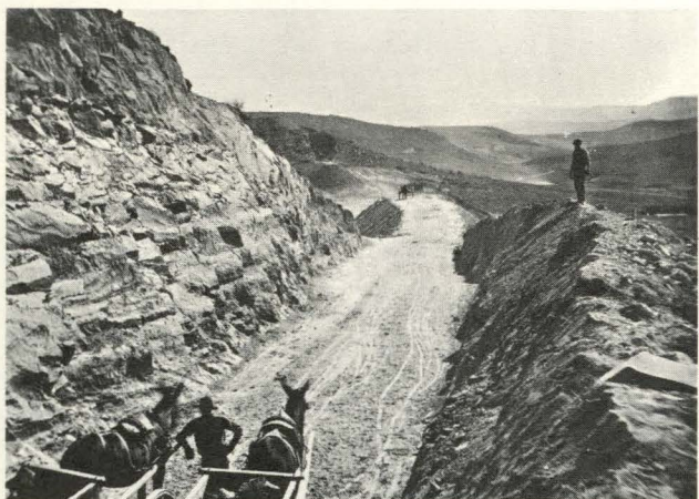
Fill work at Bitter Creek. Through Wyoming the hills had to be cut down and the valleys filled in. Fills were built from both sides of the valley at once as this picture shows.
