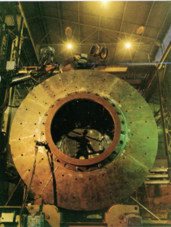
A grinding mill shown under construction in Pennsylvania will be installed during 1977 at Rocky Mountain Energy's uranium mine-mill complex at Bear Creek, Wyo. This equipment will grind 1,000 tons of ore per day.
