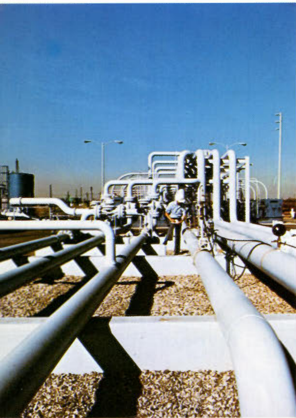
Champlin's two high-pressure water injection plants at its major Wilmington, Calif. oil field aid in secondary recovery operations. The facilities can pump 700,000 barrels of water a day into oil-bearing formations to help force oil to the production wells. Waste water is processed and recycled.
