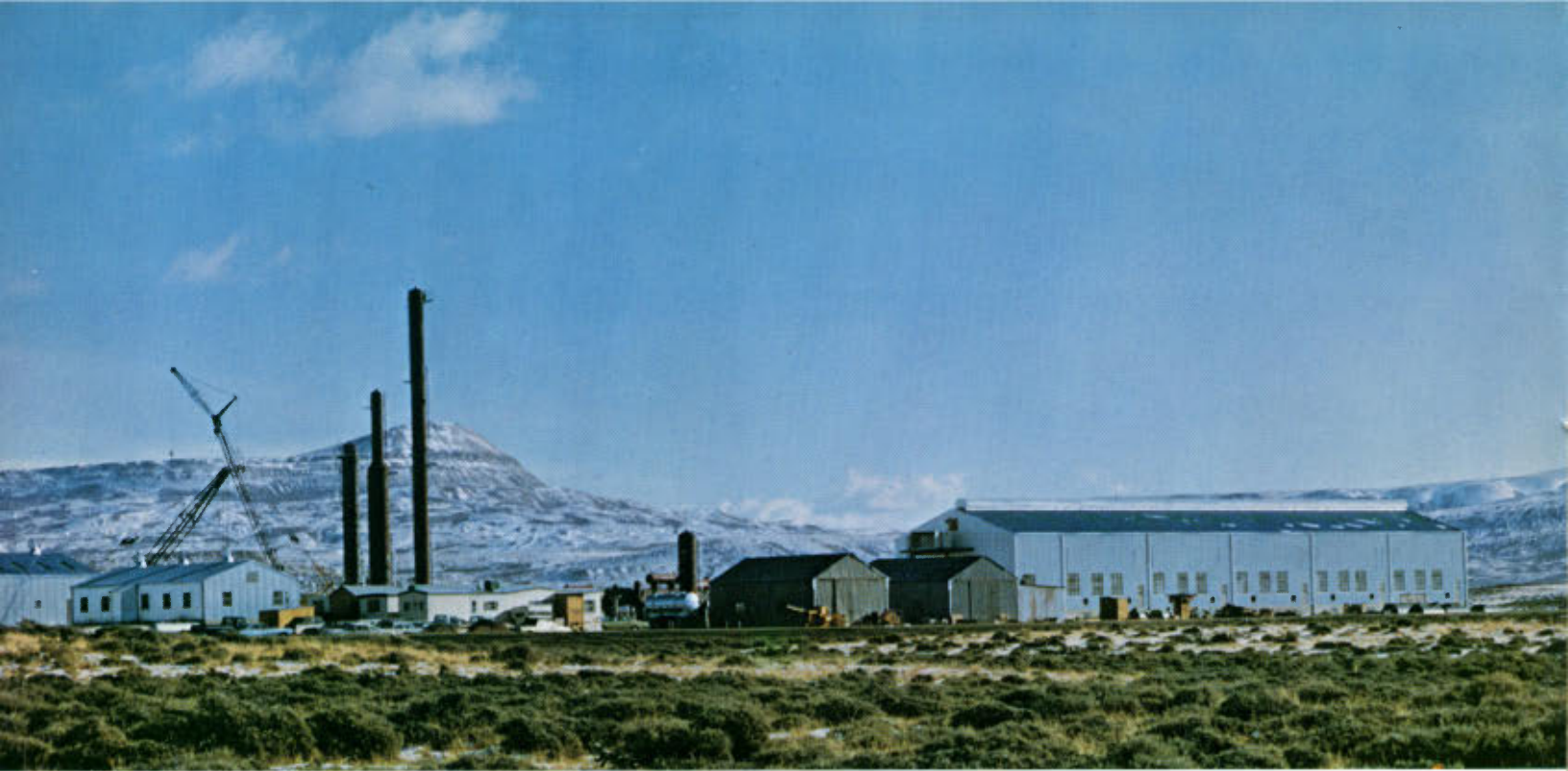
Construction of the new gas processing plant at the Brady Field in Sweetwater County, Wyo. is on schedule. Oil recovery from this plant, expected to go on-stream in August, 1975, will be transported in Champlin's pipeline.
