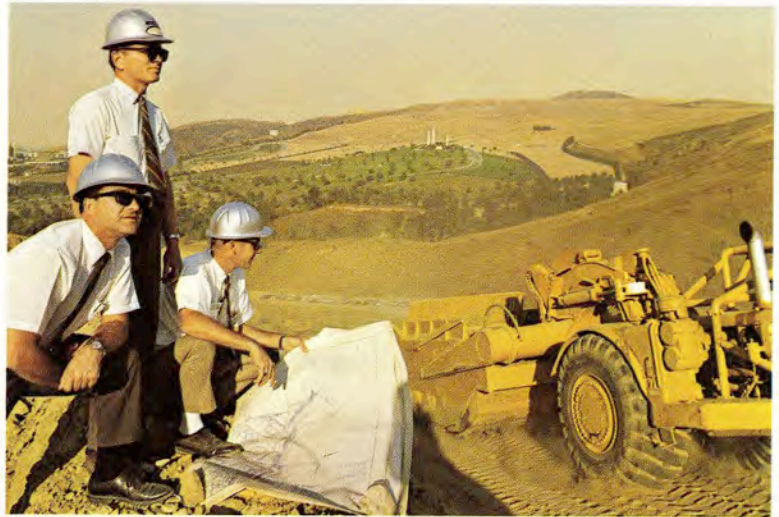
Engineers inspect grading operations at Upland Industries site for residential homes in California.
