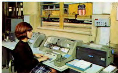
Complete Operating Information (COIN): Console operator (above) on West Coast reports freight movement data to computer center (below) halfway across the continent in Omaha.
