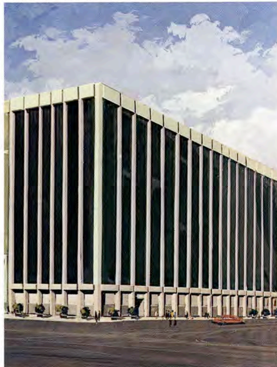
Modern, 12-story addition to Union Pacific's railroad headquarters in Omaha, Nebr., to be completed during 1971.
