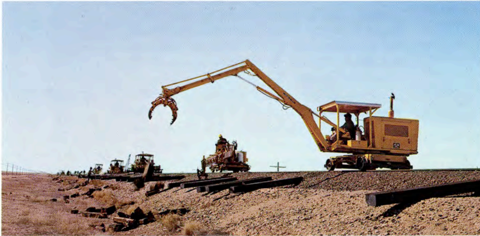
Below—Mechanized tie replacement in western Utah.
