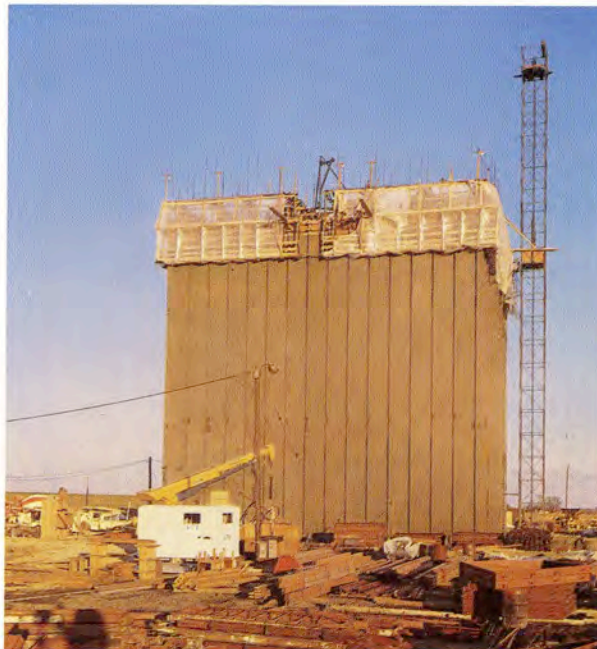
A new General Foods Corporation plant under construction at a Union Pacific-served industrial site in Topeka, Kans.
