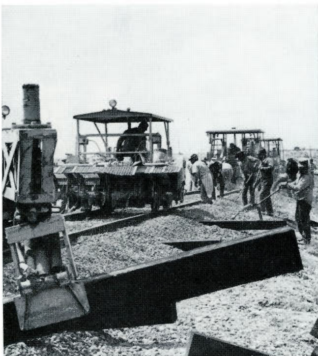
Track gang working with diversified roadway machines.
