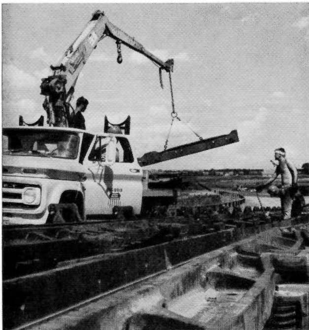
Retarders being installed in new yard at North Platte, Nebraska.
