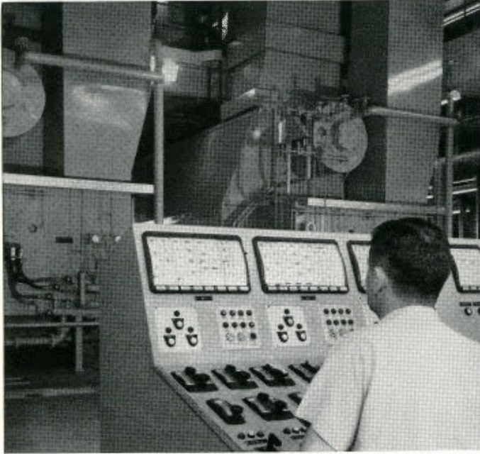
At the controls in automated power plant at Omaha.
