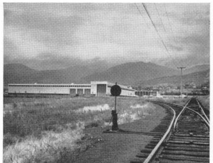
General Motors warehouse in North Salt Lake Industrial District.
