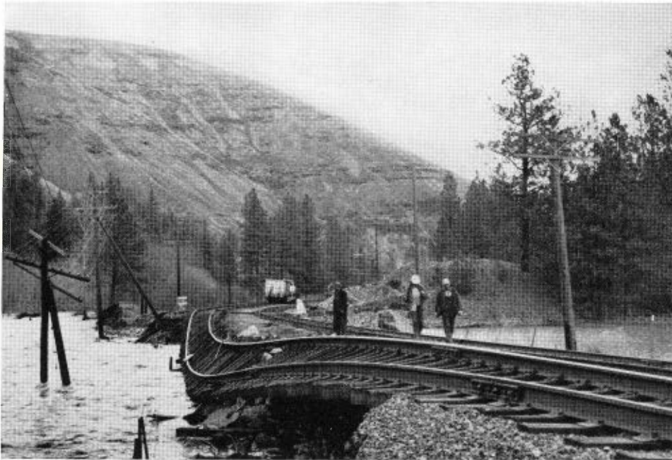
Flood damage at one point on the main line along Meacham Creek, in Oregon.
