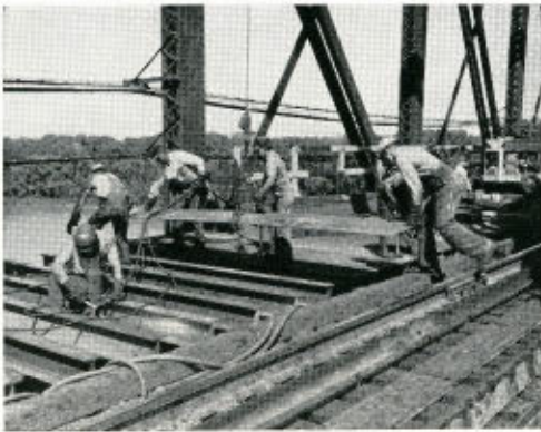
Improvement work on Missouri River Bridge.
