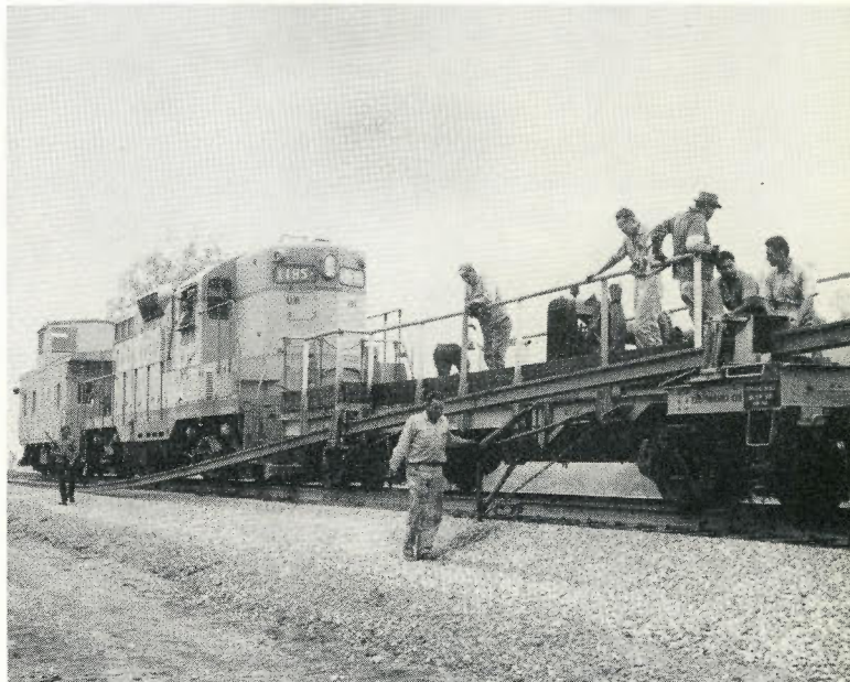
Laying welded rail between Ontario and Riverside.
