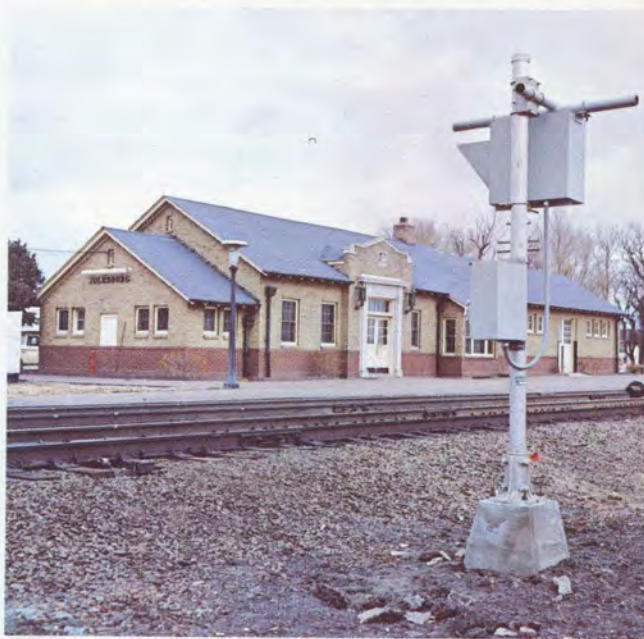
The new scanner is located just west of the Julesburg station and scans the plates on all eastbound traffic.
