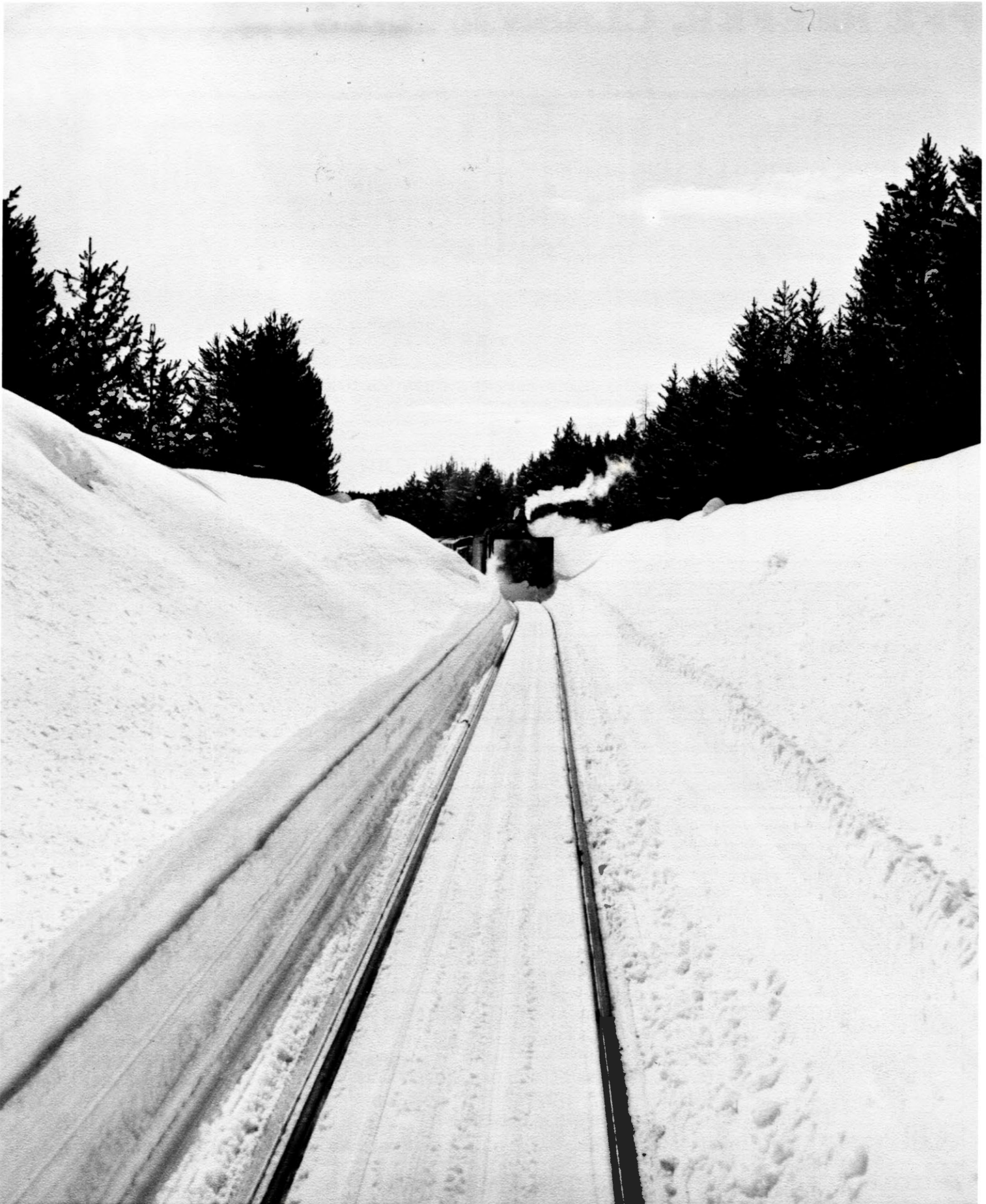
11 As Rotary Snow Plow 075 backs up to show the 'cut' made by the plow one of the Union Pacific photographers takes the opportunity to put it down on film. Photo courtesy Union Pacific Railroad.
