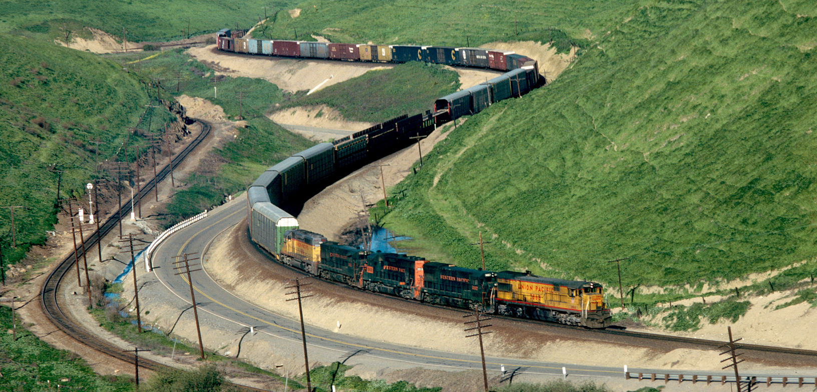
Powered by a mixture of UP and WP units, Western Pacific symbol freight APUP (Auto Parts Union Pacific) brings the Ford auto parts empties up the west side of Altamont Pass on March 18, 1980. Traffic to and from Northern California has been critical to UP's welfare since the railroad was built. As illustrated in this photo, UP played a strong role in defining the operations of SP and WP, even before the mergers. —Rob Leachman photo
