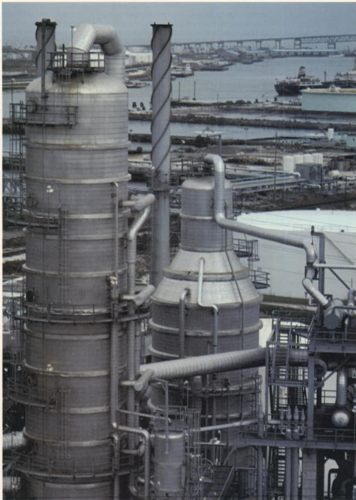
Champlin's refinery located beside the ship channel at Corpus Christi, Texas can process more grades of crude oil, including high-sulfur oil, as a result of a $250-million expansion. The crude fractionator and vacuum unit towers shown (left to right) are used in the initial stages of the refining process.
